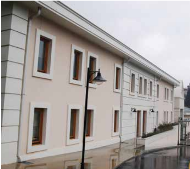
"KOC UNIVERSITY" ISTINYE CAMPUS MBA BUILDING
