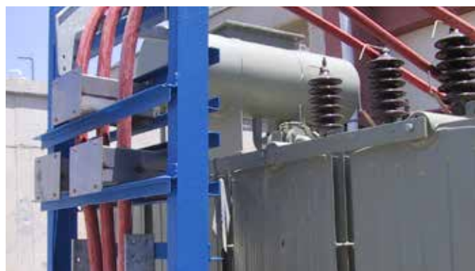
PETKİM ALİAĞA PETROCHEMISTRY COMPLEX HDPE PLANT
