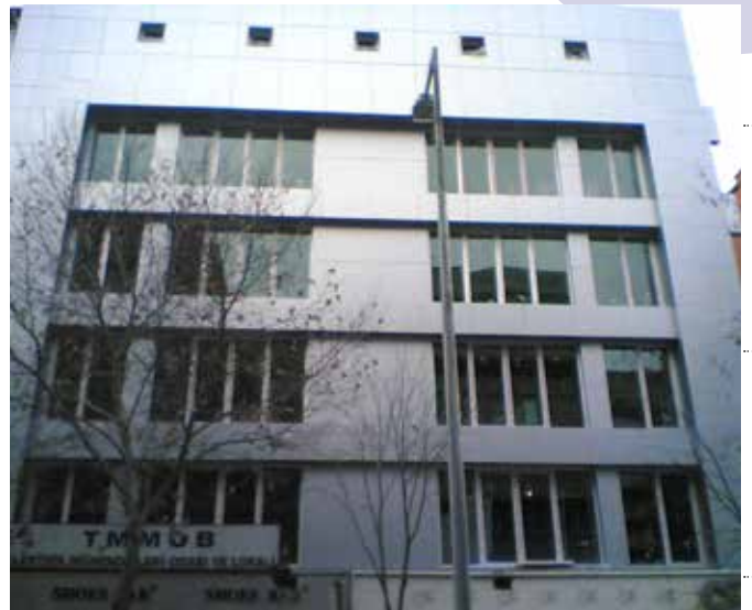
THE HEADQUARTER BUILDING OF THE CHAMBER OF ELECTRICAL ENGINEERING
